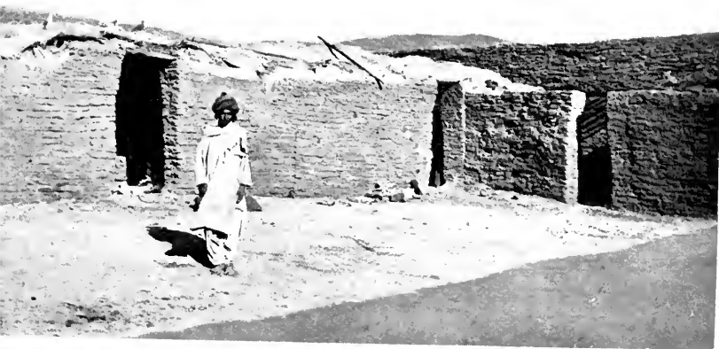
INTERIOR OF REST HOUSE, MUKAK.
